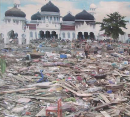
Debris at main mosque in Banda Aceh
